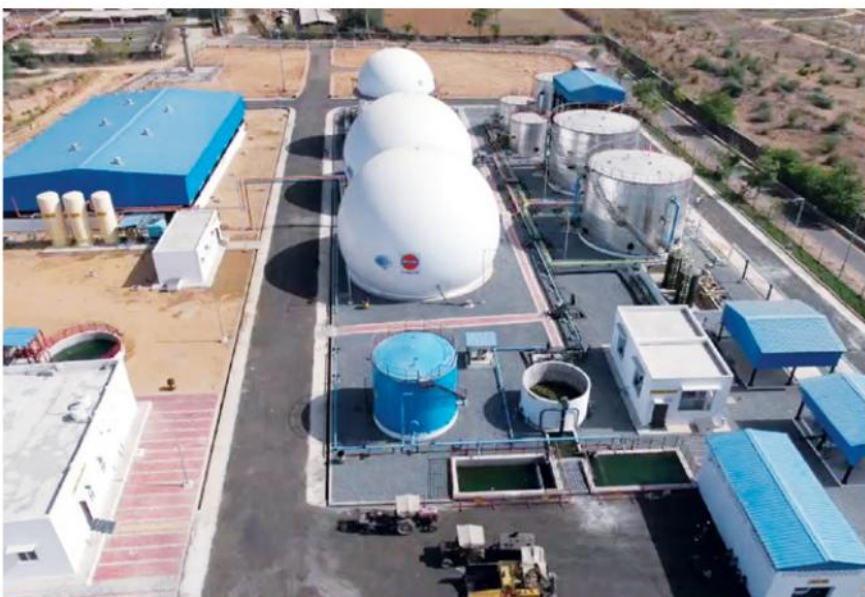
CBG plant at Hingonia, Jaipur
