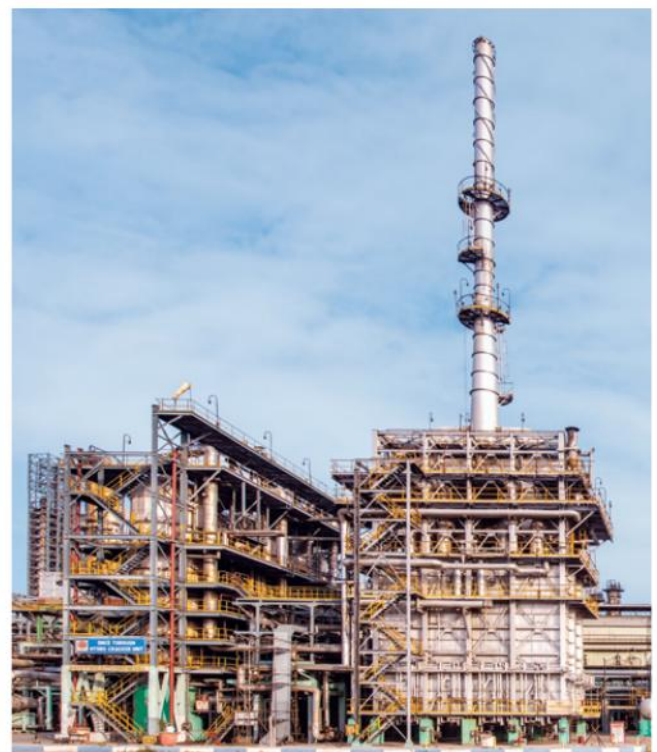
Hydrocracker Unit at IndianOil Panipat Refinery
