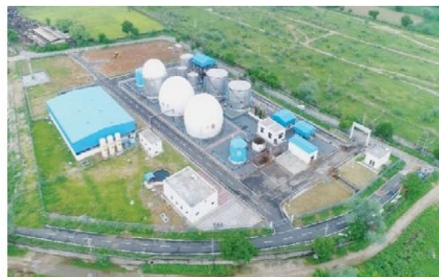
100 TPD Compressed Biogas Plant at Hingonia, Jaipur
